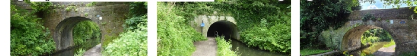
⑤ Bridges on the Peak Forest Canal - Grade 2 Listed
