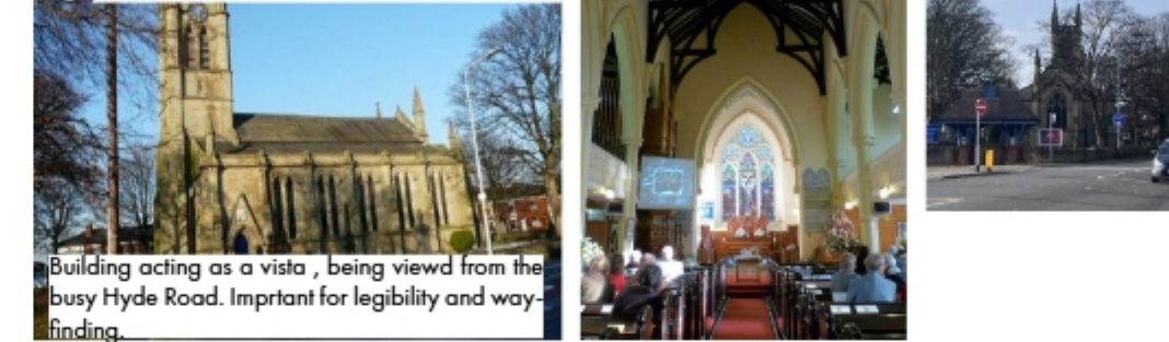
① Church of St Mark-Grade 2 listed
