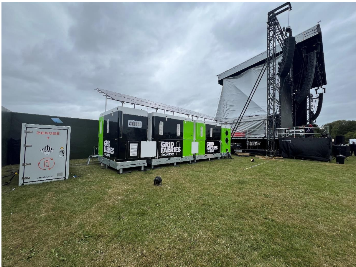
Image 1: Battery system for main stage
