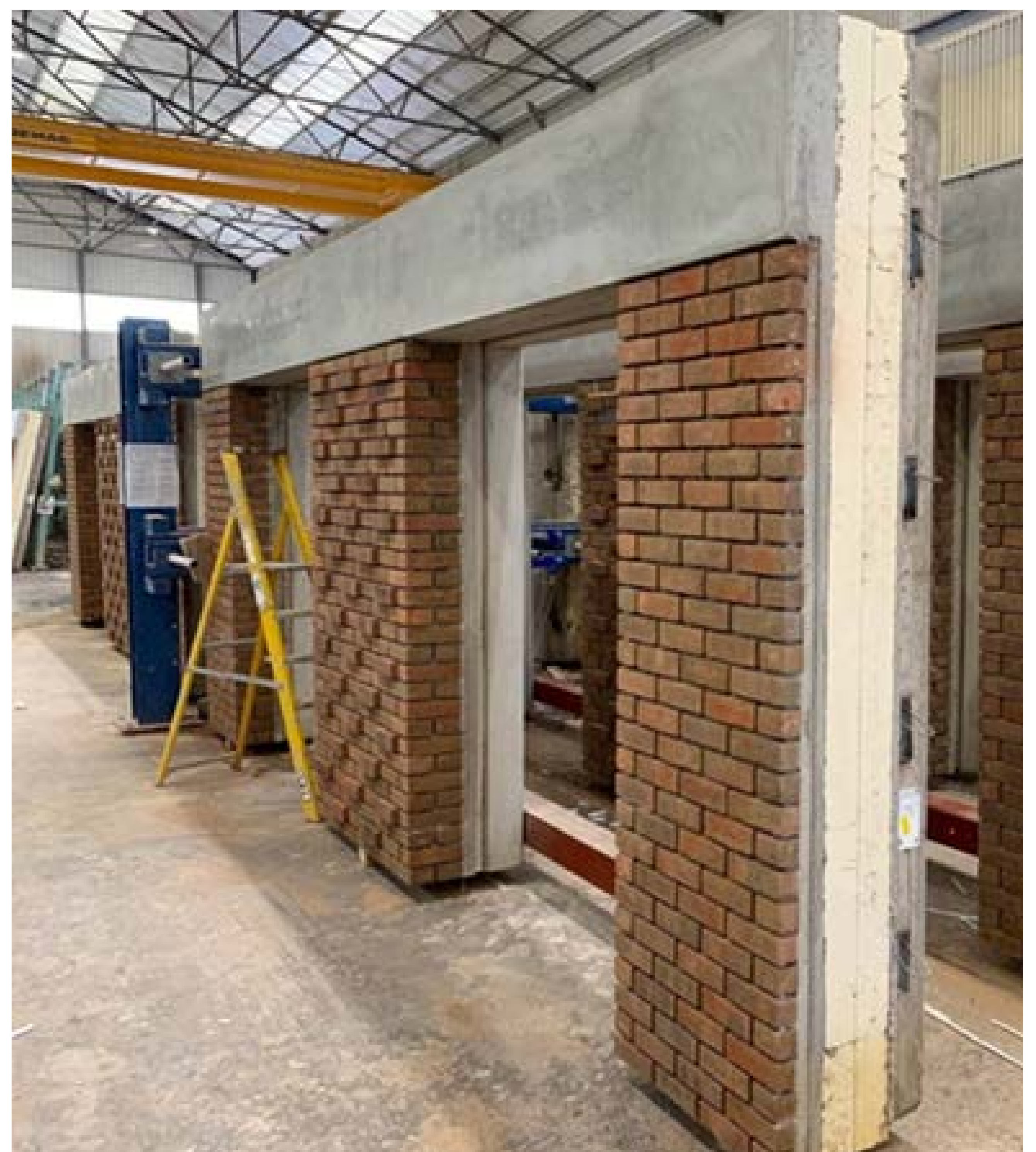
An indicative example of modern methods of construction within a factory environment. Panels are produced in factory conditions, which significantly reduces the carbon footprint of construction projects
