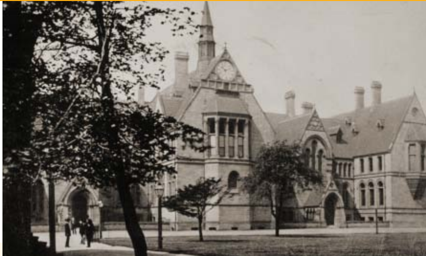
Early shot of John Owens Building
