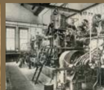
Experimental engines in the engineering laboratories
