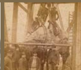
The excavation of the boulder that sits outside the Beyer Building
