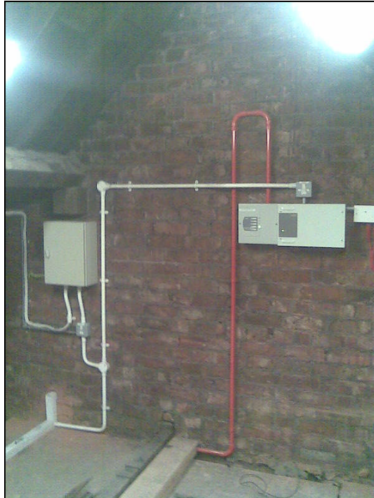
Photograph showing modern fire panel in roof void above 3.04 where University of Manchester employees or contractors may need access
