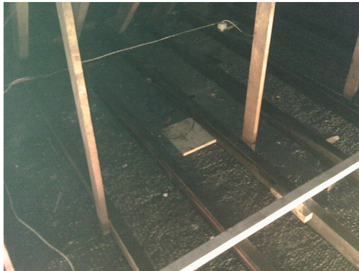
Photograph showing exposed plaster and wiring conduits in roof void above Room 3.03
