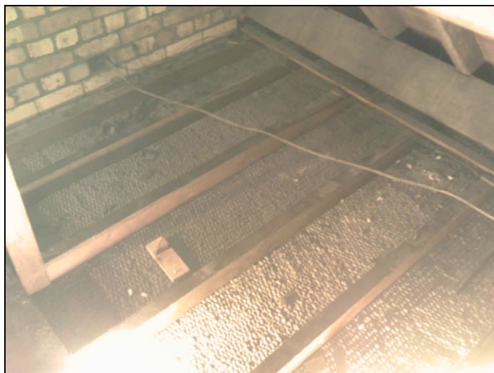
Photograph showing exposed plaster and old wiring within roof void above room 2.53
