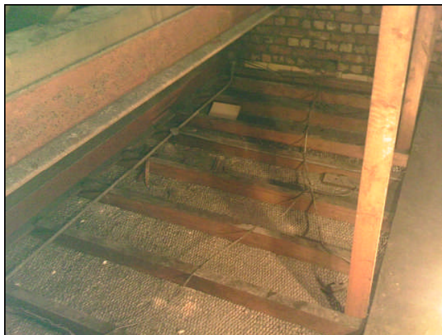
Photograph showing redundant cables RSJ within the roof void above room 2.54.
