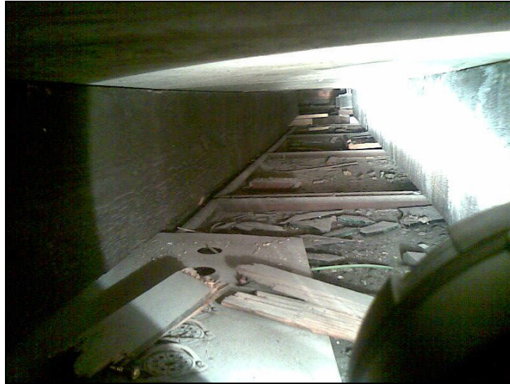
Photograph showing debris under suspended floor in roof void above Room 3.04
