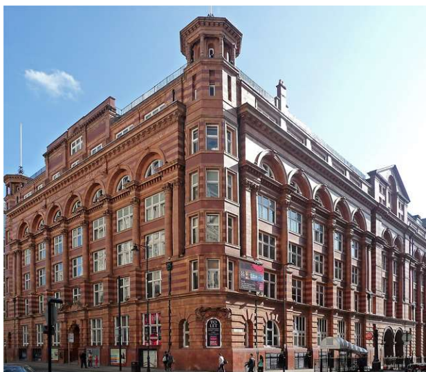
The Tootal office building in Manchester, where I was able to carry out my internship
