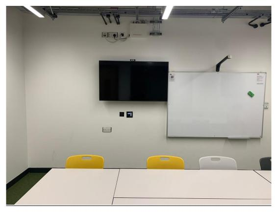
The lecture capture device is enclosed in a plastic case above the teaching monitor in each of the 10 and 20 seater rooms.
