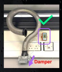
Once the air flow is at the correct velocity, the indicator will display an arrow and the LED will stop flashing.
