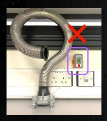
The air flow indicator will display a cross and the LED will flash until the damper is opened.
