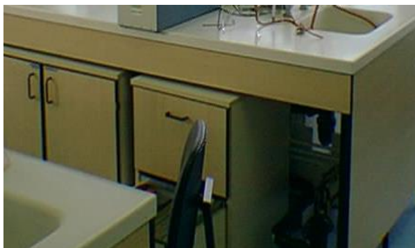
Laminated under-bench storage cupboards mounted on castors to facilitate cleaning
