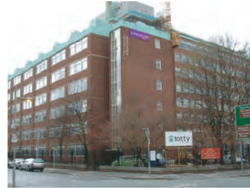
Sign 16 (Tray Sign and Letters) Chemistry Building
