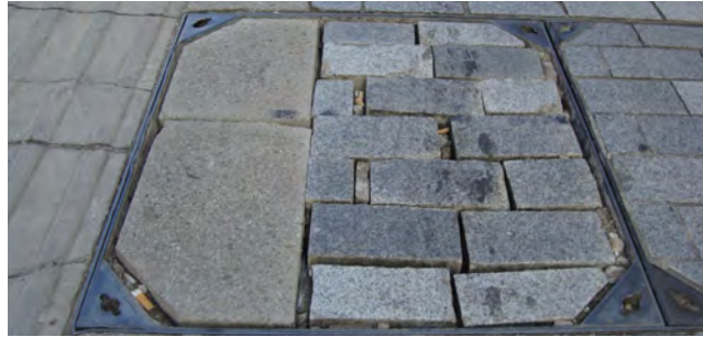
Paving failure in recessed cover
