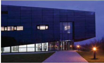
Dalton Cumbrian Facility
